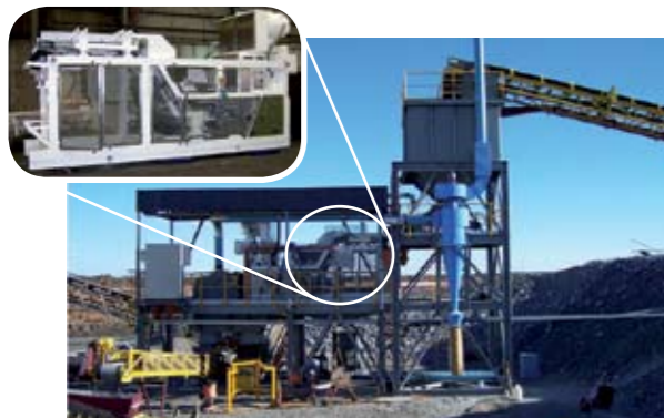
UltraSort UFS-EM installation at Consolidated Minerals Kambalda Operations, Australia.
